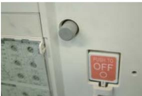
On the manual reset type (optional), the gray manual reset button on the front side of the breaker will stick out to continuously output OCR alarm (AL) if the breaker is tripped by the electronic trip relay. After tripping, the breaker can not be turned on unless the manual reset button is pressed for resetting.
